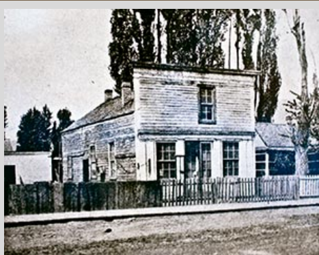
Smith broke into this building in 1865, stuffed territorial papers into saddlebags and escaped to Washington Territory with a U.S. Marshal on his heels. Photo courtesy: Nez Perce County Historical Society, Ira Dole collection
